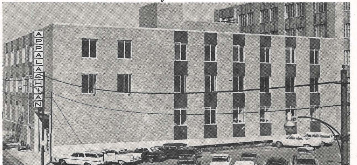
Sparkling new, and ready for occupancy as October began is the 40,000 square-foot addition to the general office building in Roanoke. The big door at the rear is a covered loading dock; the sidewalk covers imbedded cable to melt ice and snow, and the interior colors are bright, different, and cheerful.
