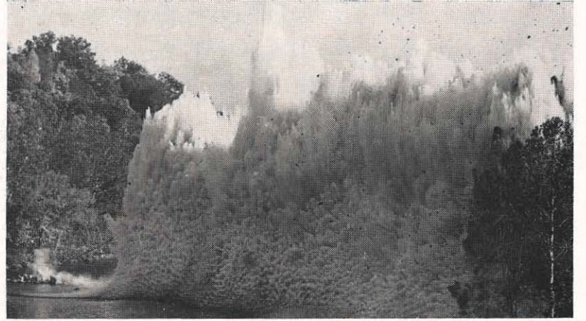
This is what the James River looked like as a blast of 3,300 pounds of dynamite had ripped the river bottom. A trench had to be dug to accommodate an oil pipeline, located 150 yards below Reusens hydro plant. The shots were laid in 57 holes, and fired at intervals of 17 micromillseconds apart to reduce concussion and shock to the dam.
