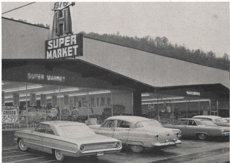
This two-unit shopping center owned by brothers has become Charleston's newest all-electric commercial facility. The building, heated and cooled by heat pumps, covers 9,600 square feet; half is given over to super-market operated by Orville Haynes, the other half to a hardware store operated by his brother Vernon. The total connected load for both is 155.8 kw.
