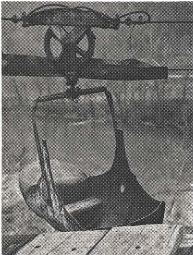
Company men whose jobs send them out into less-traveled areas see a lot of odd things, but few as odd as this aerial chair lift across the Coal River in the Charleston division. The rider climbs aboard, the operator plugs in the motor, and the chair goes over the river 40 feet below. This lift has been in operation for 20 years, but it hasn't always been electric.
