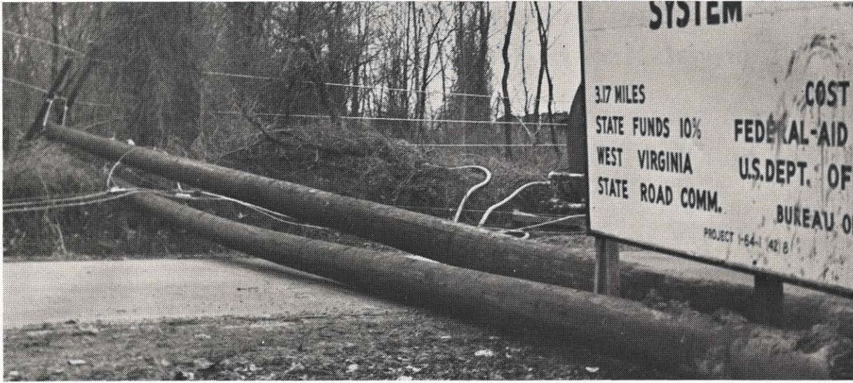
The Huntington division lost a pole recently, and the way it happened was right out of the pages of science fiction. A new stretch of line had been installed, and on it the telephone company put its lines. A push brace was added to one pole for further strength; early one morning this pole began to rise like a rocket off the pad; it was restrained for further
