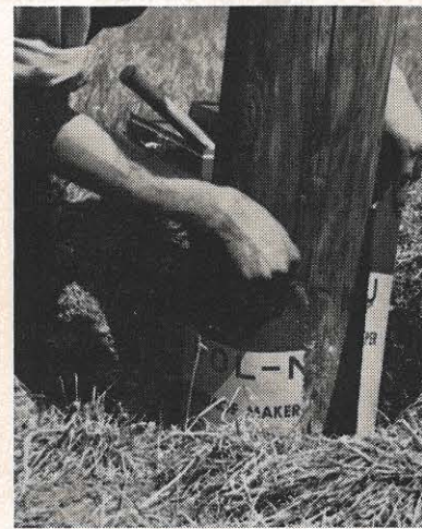
last step is filling and tamping the hole.
