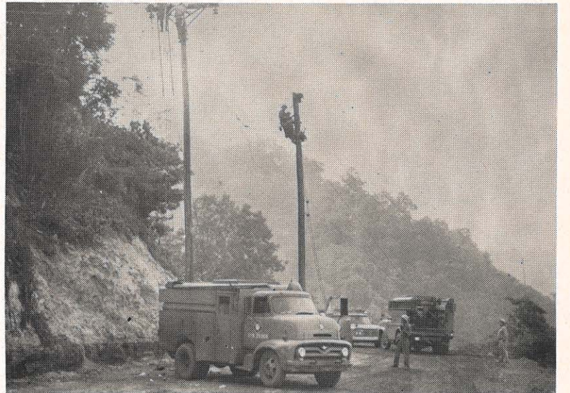
M. K. Spraker's crew is busy replacing a pole on a line serving a new mine in the Bluefield division. On the first pole are Mr. Spraker and Walter Thomas; on the second, H. S. White and John DeBusk; on the ground, John K. Morgan and G. E. Adams.
