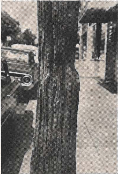
Many things can happen to electric service poles, from lightning to woodpeckers. Somewhere in between is the Great Bored Youth, who finds it amusing to whittle on any pole located in front of a drug-store, like this one in Roanoke.
