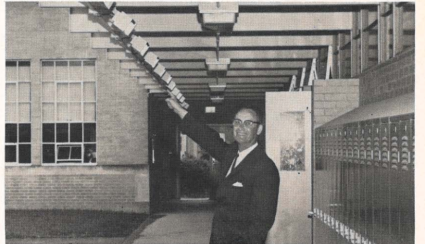
A happy Jim Wyson, Huntington commercial sales representative, points to the solution of the question, "How to heat electrically, outdoors."
