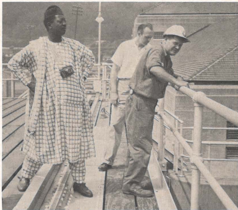
Kanawha River locks are inspected by Emanuel Aileru, assistant director of inland waterways in his country's Ministry of Transportation. The Nigerian, in native dress, was shown the power generating facility by D. E. Sayre, Huntington Corps of Engineers, and G. V. Loveday (in hard hat), Marmet hydro plant utility operator for the Kanawha Valley Power Company.
