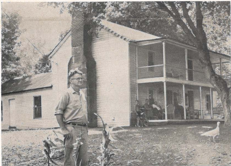
Striking the pose of a country squire in front of his century-old house is M. T. Miller, retired Charleston truck driver-groundman. His retirement project is nothing less than the complete renovation of the place. The chimney, visible behind him, was originally made entirely of the huge stone blocks in the lower half; over the years the top blocks were replaced by brick.
