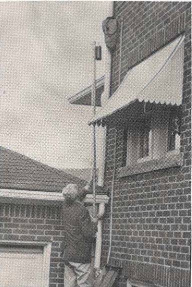
Tip Fletcher, line inspector in Bluefield, knocks out a nest of hornets with a can of pressurized insecticide ingeniously mounted on a specially-equipped hotstick. Hornets and similar creatures often make their homes around service entrances.
