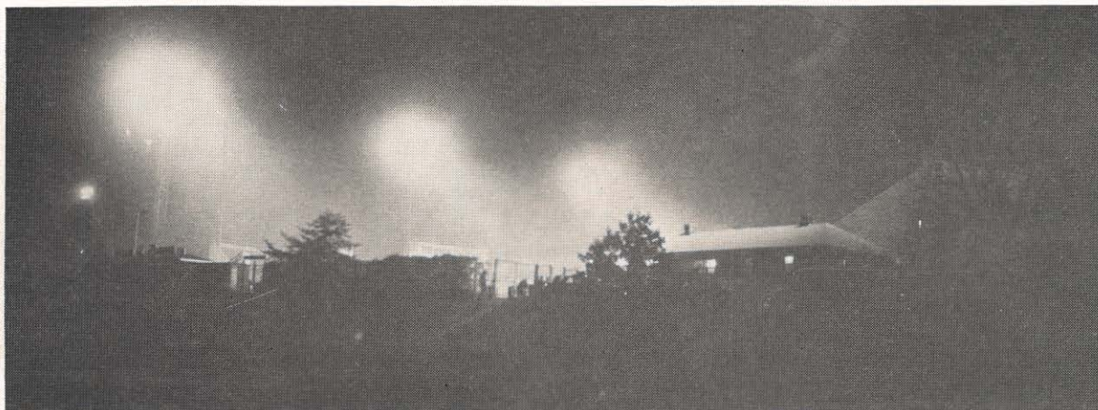
When there's activity at Bluefield Stadium, everybody knows about it, because the sky is brightly lighted above it, thanks to a new lighting system just installed. Three 80-foot light towers on each side of the stadium were set in, each tower carrying 36 1500-watt flood
