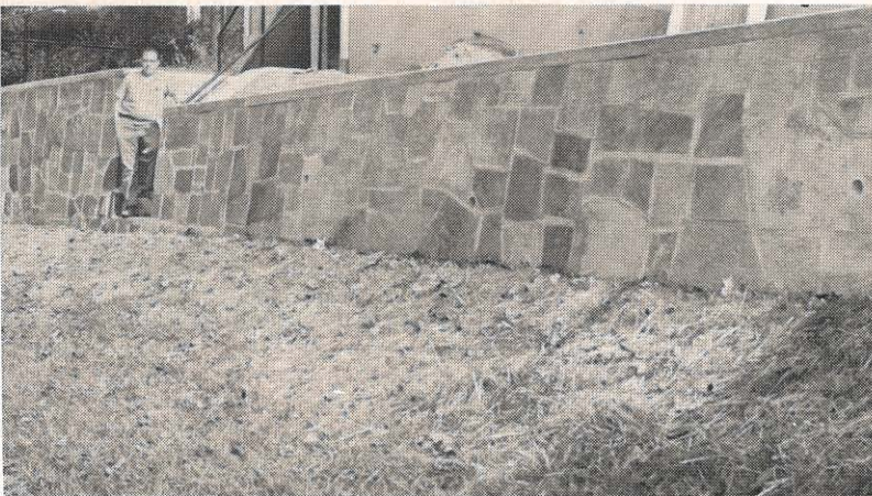
Shown here is a portion of a 61-foot-long wall J. B. Rhudy completed at the rear of his home at Welch, after three years of do-it-yourself work which included hauling thousands of stones, mixing 96 bags of cement and 17 tons of sand, and countless man-hours of his labor.
