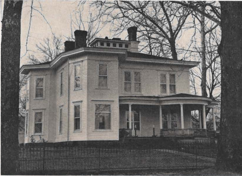
This house, built in 1853, has recently been converted to electric heat, all 17 rooms of it. Its first owner was one of those who voted for statehood for West Virginia.
