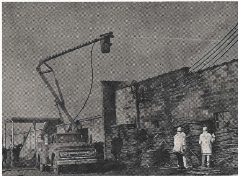
Up above the smoke and flames in an Appalachian bucket truck, an Abingdon fireman plays a hose on a major fire in that town last month. The truck was pressed into service when the fire, already big, threatened to spread.
