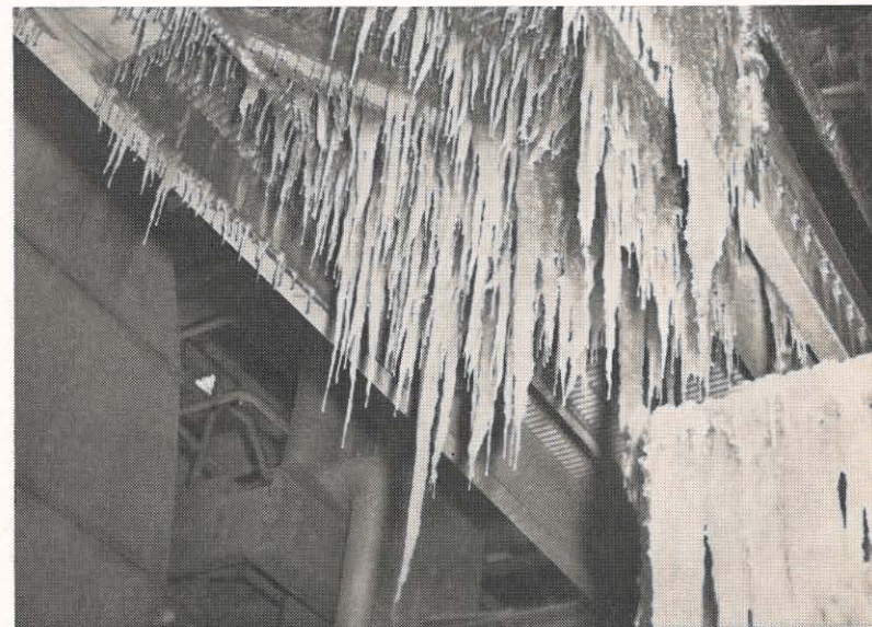
Maintenance work performed during a recent outage at Philip Sporn plant presented certain problems, as this picture shows. The work was done on Unit 5, an outdoor unit. At ground level the temperature was seven below zero, and at the top fan floor, it was 20 below. Portable heaters and windbreaks protected the men from the weather.
