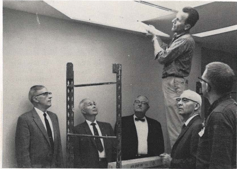
Interested in the progress of the remodeling of their old headquarters, a group of retired Charleston employees dropped in for an inspection tour of the office building. Leo Yon, center, contractor's superintendent, explains the lighting layout to Ray Dixon, Hobart Ballengee, Ira Gillikin, and O. L. Williams. That's Bob Lowther, building supervisor, with his back turned.
