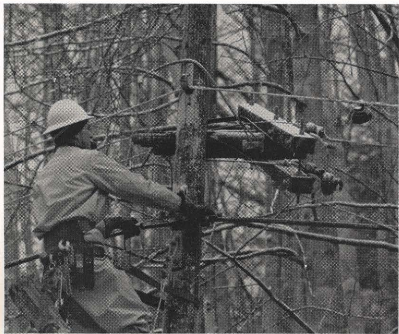
Buttoned up against the intense cold, a lineman works to restore service after an ice storm took out lines and poles in the Roanoke area. (Roanoke Times photo.)
