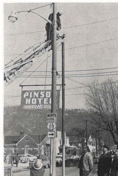
The last incandescent fixture in downtown Pikeville comes down. Charles Ratliff is the groundman, Homer Helvey the lineman, and Jesse Collier the working foreman. Pikeville's city manager, W. E. Butcher, and H. H. Kincaid, division manager for Kentucky Power, watch at right. The city's entire street lighting system was converted to mercury vapor.
