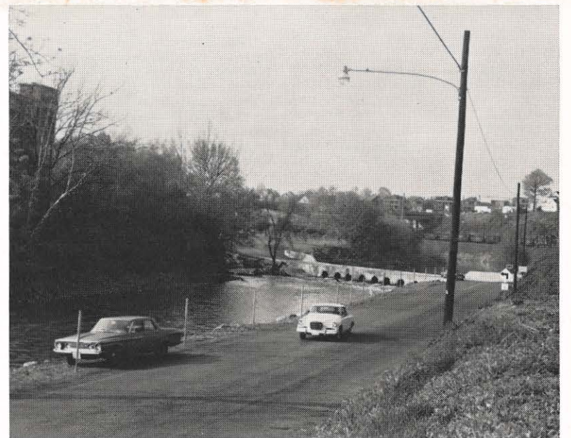
Twenty-four 10,000-lumen lights have been installed along Roanoke's scenic Wiley Drive. Nearly a mile long, the drive twice crosses Roanoke River, and connects South Roanoke Park with the city's Transportation Museum. Along it the city has planted grass and trees and installed picnic benches and outdoor fireplaces for cooking. Future plans call for the extension of the river-side drive all the way to Salem.
