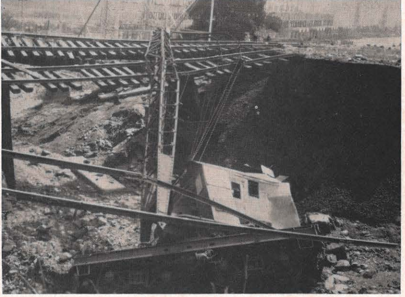
It was 30 years ago that cloudbursts and a flood on the New River knocked Glen Lyn plant out of service for a month. This shows what the plant was like after the flood had passed. To clean ashes and debris out of the plant, it was necessary to hire 300 temporary employees, and it was three months before the plant and plant area were restored to normal conditions. The Monroe Watchman recalled the flood in a recent issue, and prompted Glen Lyn's Ed Jones to send this photograph.
