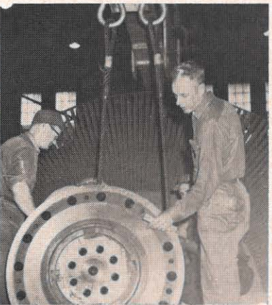
For the second time in 21 years the rotor in Glen Lyn's Unit 5 has been changed. R. B. Comer and D. L. Garrison balance the turbine rotor during the recent major overhaul on the unit. At one point in the unit's life it was operated for more than 27 months without being taken out of service.
