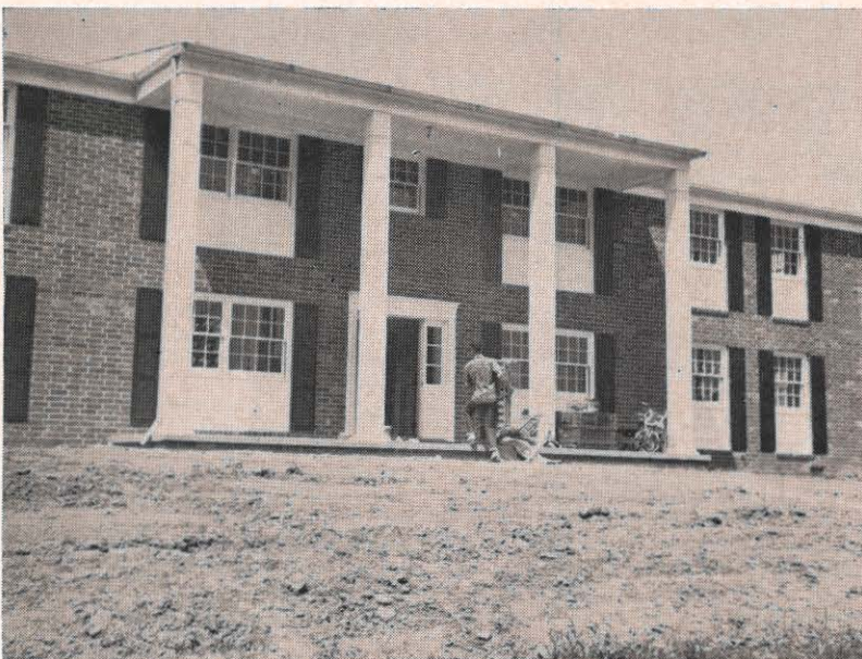
While some units are still under construction, and some streets still not paved, the total-electric Monticello apartments in Abingdon have already begun to exert their appeal. Here movers carry the first tenant's possessions into a new apartment. The project has 18 units.
