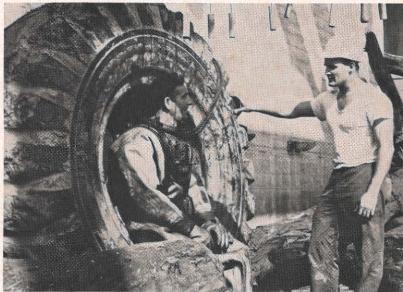
Maintenance work continues on the Marmet, Winfield, and London hydros on the Kanawha River near Charleston. Here, Diver Sam Whitson relaxes in a giant tire he found while inspecting rack bars, and talks to Jack Jarrett, mechanical maintenance man. The tire and the tree trunks are just part of the debris he found at the bottom of the river. He also recovered four pontoons lost last year. Winfield and Marmet hydros were also painted after nine weeks of sandblasting. Used were 305 gallons of subway black and 150 gallons of stainless steel paint.
