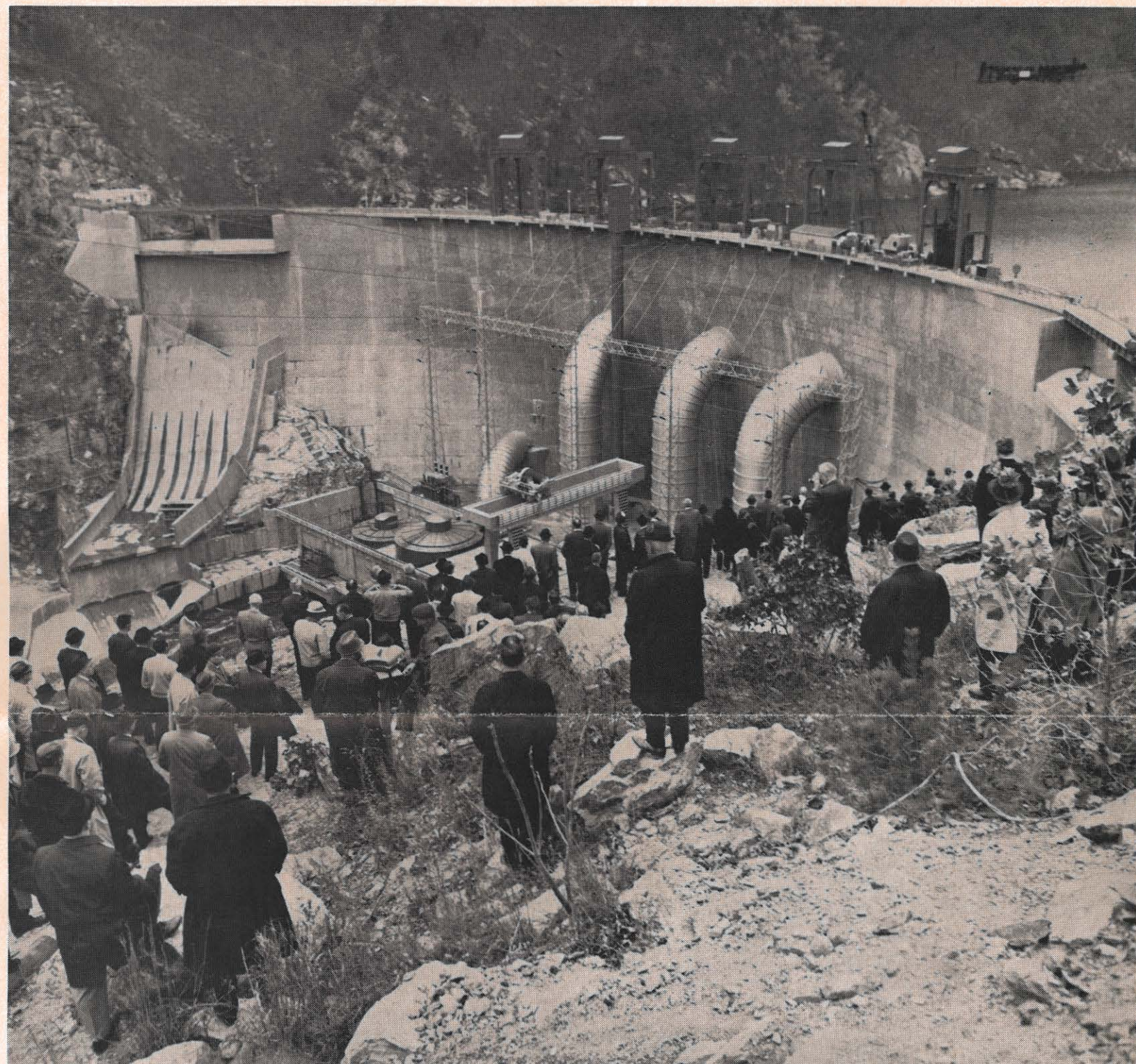
Appalachian Power Company's Smith Mountain Project, on the Roanoke river 45 miles southeast of Roanoke, was visited by approximately 300 management personnel Wednesday, November 10. The trip, made in nine chartered buses, included a tour of the powerhouse, where the upper dam's four generating units are located, an over-all view from the proposed overlook area, and a stop at the Haleford Bridge 12 river miles
