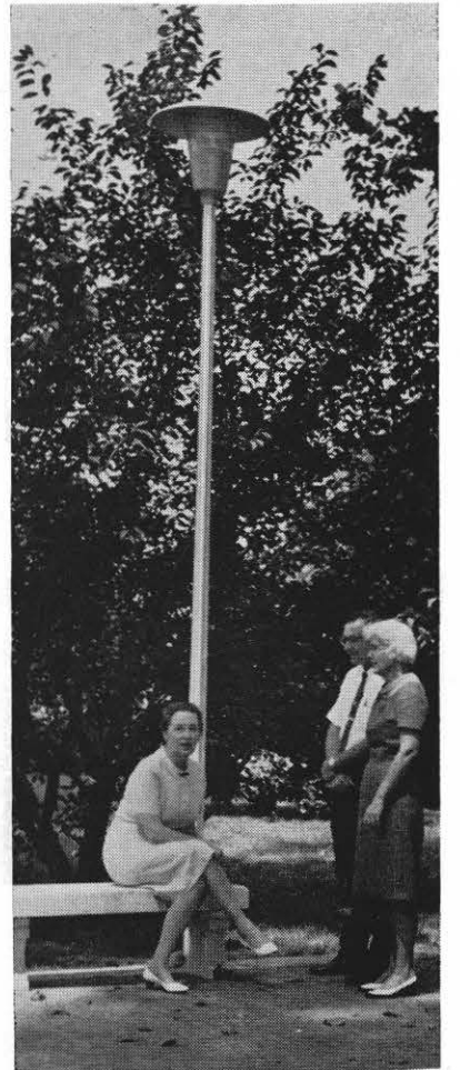
Historic Ruffner Park in Charleston got a bright new look recently, thanks to the efforts of the Kanawha Garden Club. Seeking to reduce vandalism in the area, the group campaigned for, and got, six 7,000-lumen mercury vapor post-top luminaires. The thanks of the group were expressed by Miss Mazie Young, park project chairman of the club, and Mrs. Turner Ratrie, president, to Kenna Judy Jr., division engineering aide, who engineered and expedited the job.
