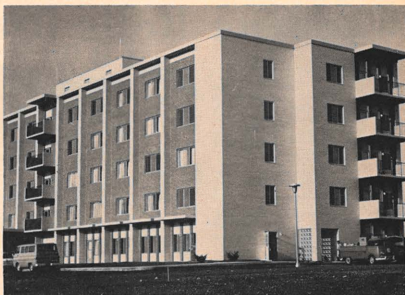
This is Friendship Manor, home for the aged built in Roanoke by the Church of the Brethren. Modern in every respect, it is total electric with a connected load of 1,200-kw.
