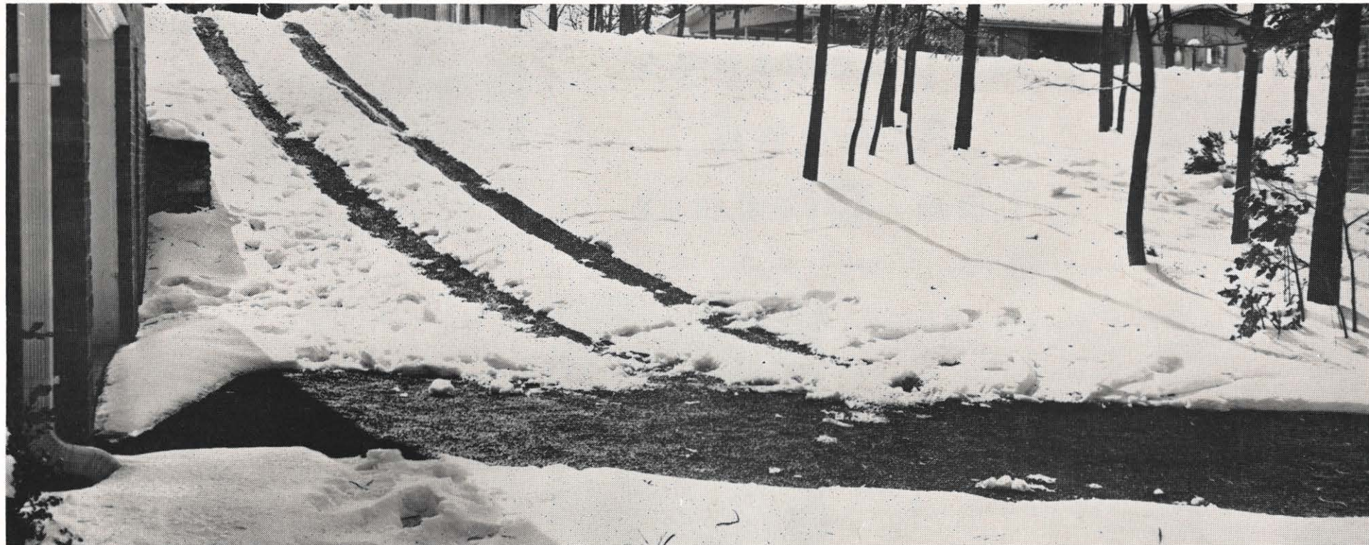
Bottom Ash-Based Asphalt Driveway Remains Clear, Thanks To Electric Heat
