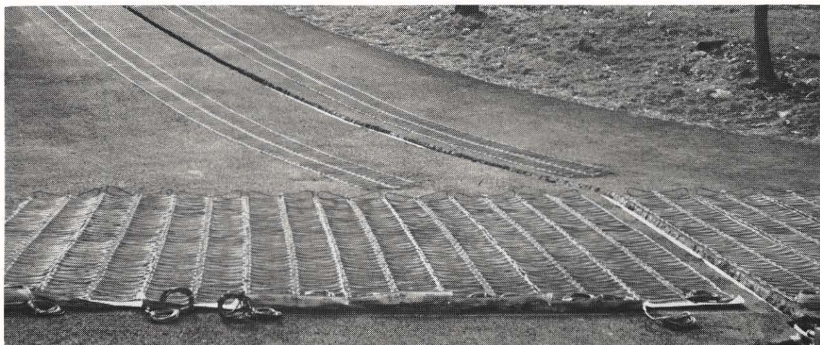
Digging in existing asphalt is required only for junction boxes and conduits (above). Electrically heated mats are placed on top of former material.
