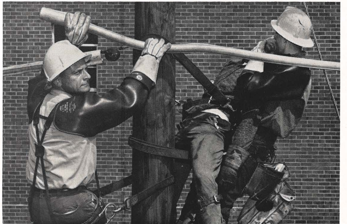
Mouth-to-mouth resuscitation and heart massage is administered as fellow lineman covers exposed conductors and relieves victim of climbing spurs and sharp objects.
