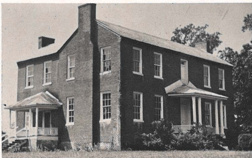
Edgemeade Boys' Ranch before the renovation started.
