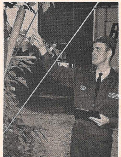
Ernie Colegrove spots clothesline on guy wire pulling shield loose.
