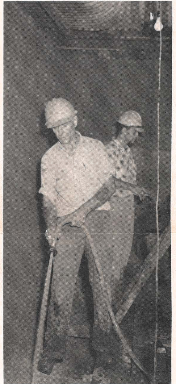
Park Sutherland (left), and Don Lasley clean up after "shooting" refractory in Clinch River's unit 3 ash hopper.
