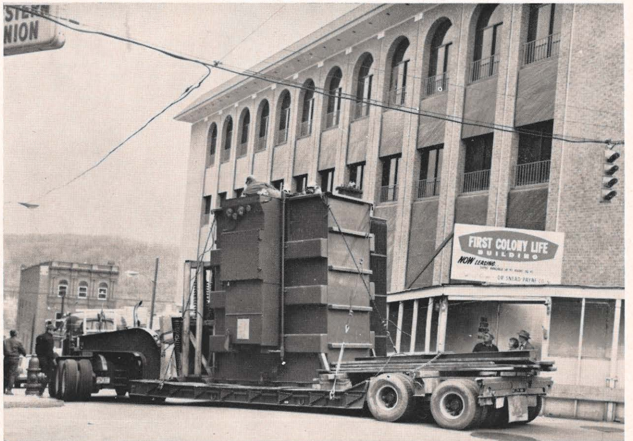
Recently it became necessary to move a 50-ton transformer through downtown Lynchburg. The transformer for the new Wright Shop Station was too large to go over the expressway. So special permission was granted by the police department to bring the equip-
