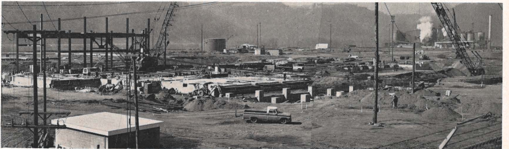
Foundations, steel structures start to take shape at Mitchell Plant site
