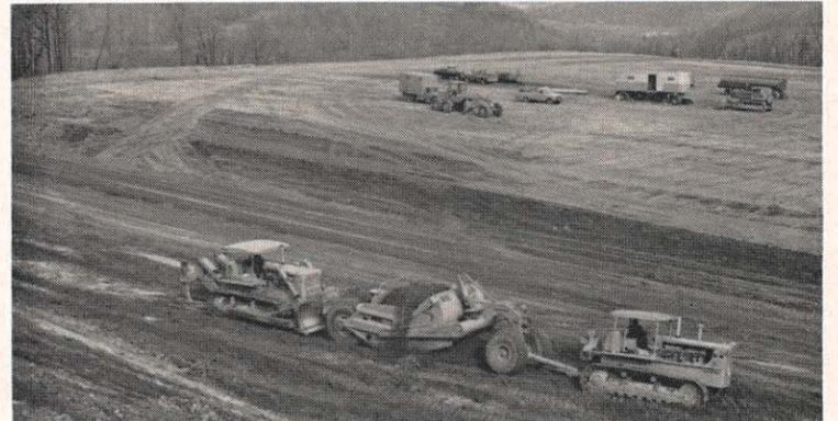
The land has been cleared for the Matt C. Funk station west of Salem, Virginia. When completed the station will be a major 138-kv and 345-kv distribution site as well as a 765-kv station. The 345-kv station area will exceed six acres and the 138-kv area will have an additional three acres. The proposed 765-kv station will be even larger. So far 109,620 cubic yards of dirt have been moved from the 345 site and 72,370 from the 138.
