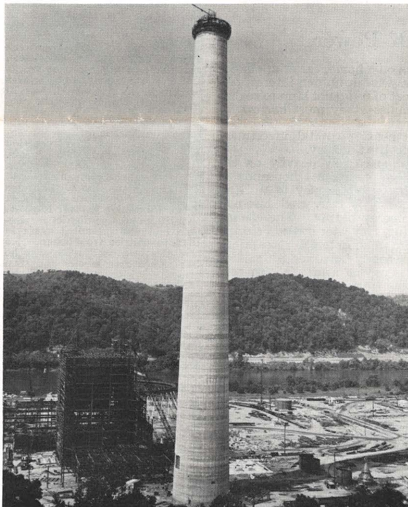
The Mitchell plant stack looks high here, but it was only about two-thirds completed at some 800 feet when this picture was taken. See "topping out" story below.
