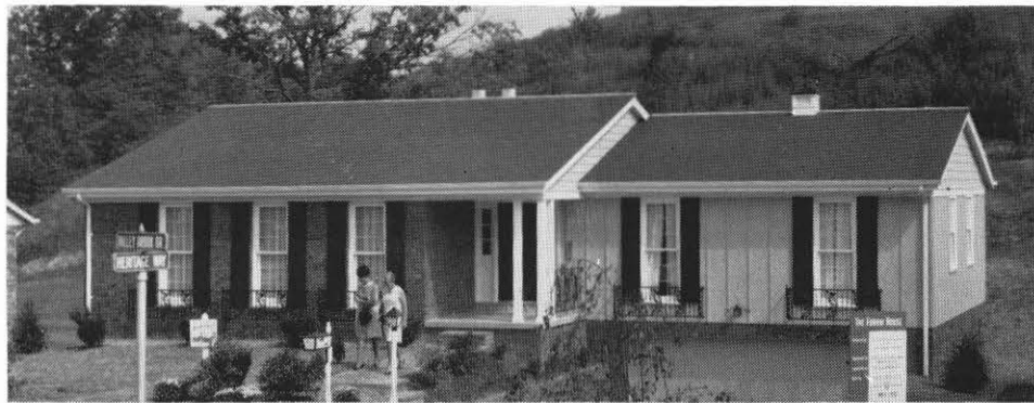
The unpretentious exterior of the Forum House is compatible with any surroundings.
