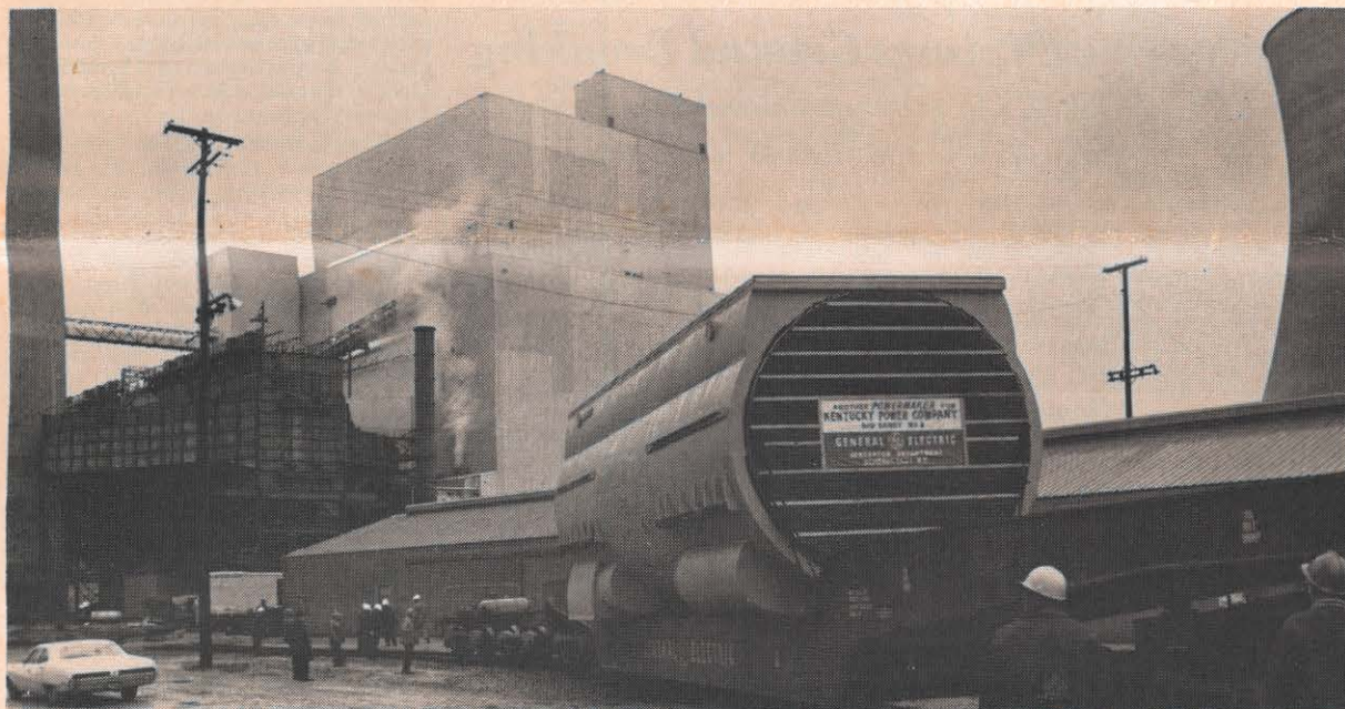
Giant Generator Awaits Equally Giant Job Of Installing
