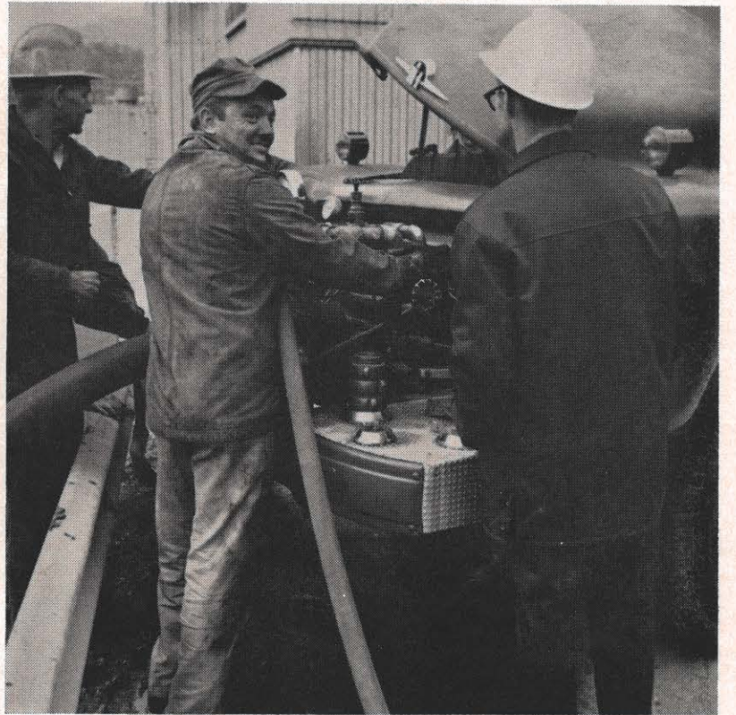
James R. Trail (from left), pump man; Edward C. Carr, hose man; and Fire Marshal Lovell H. McDonald looking at the fire pump and hose connections of the Clinch River Plant fire engine. In this particular practice, they are siphoning water from the cooling tower flume and pumping it out through the standard fire hose in the center of the picture. This procedure is used when no fire hydrant is accessible or there is a failure of the normal source of water.
