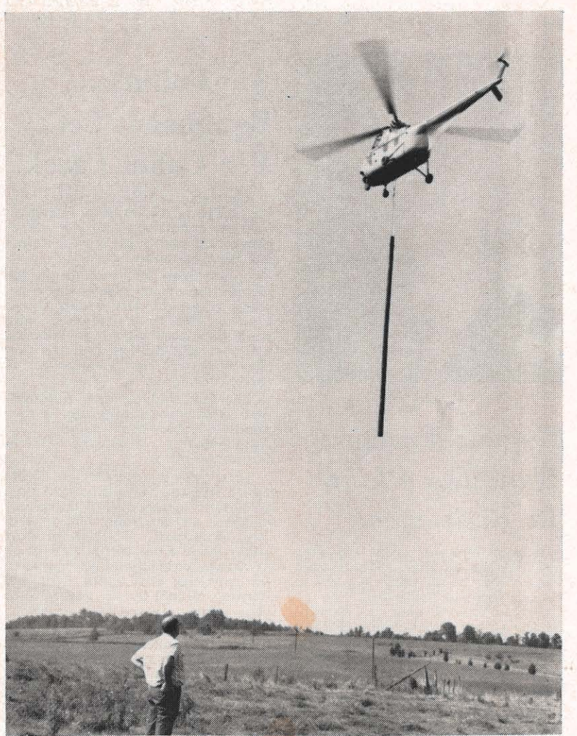
Paul Bailey, Lynchburg Division superintendent, watches as helicopter carries pole to replace one washed away in flood.
