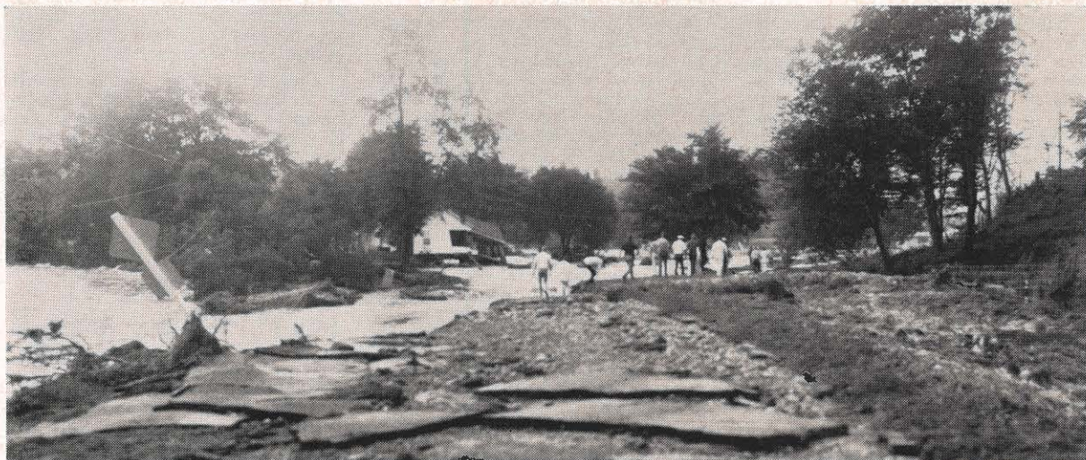
Devastating flood water receded to leave ripped up Route 778 leading into Lowesville. House in background was ripped from foundation and moved several blocks.
