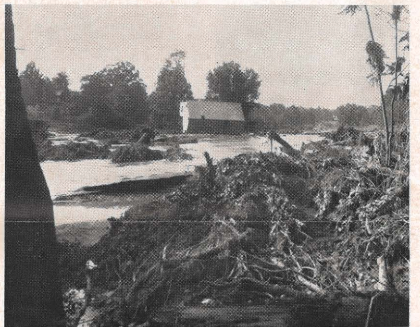
This two-story home was turned over by the water at Roseland. The Roseland Post Office building which was located next to this home was swept several miles downstream.
