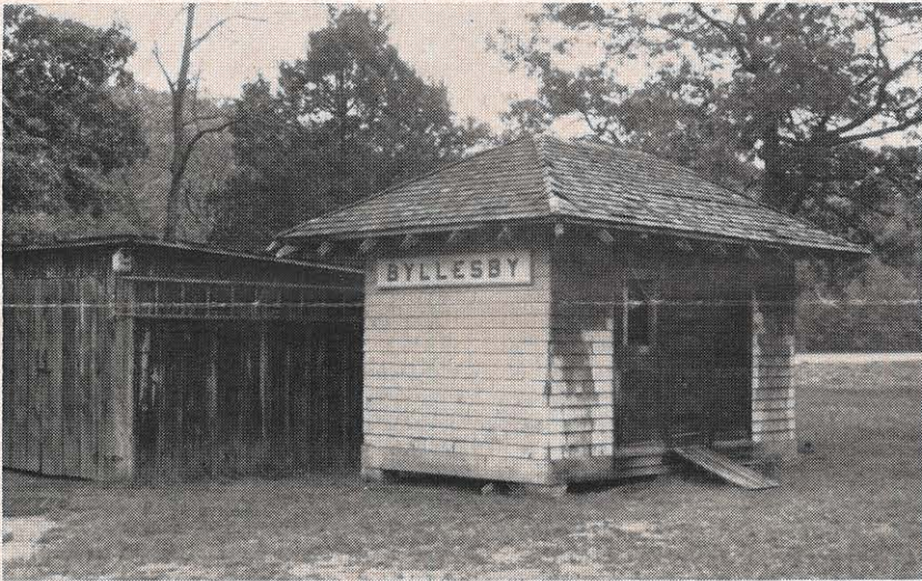
A tattered remnant of days that were—this was once the flag stop for the Byllesby Train Station of the N&W line between Pulaski and Galax.
