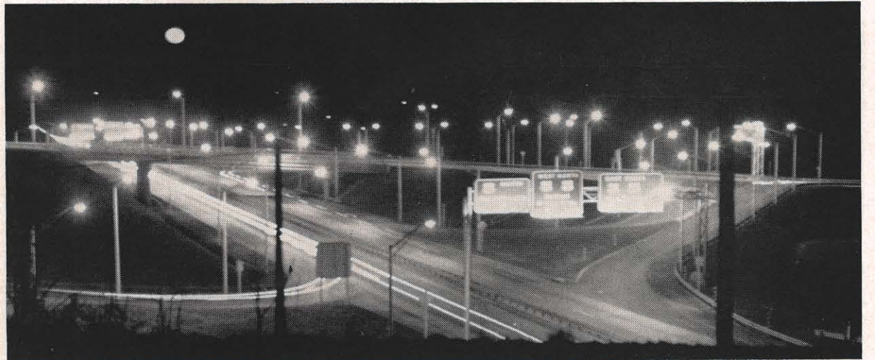
Route signs at the expressway junction of US 29, installation of Lynchburg's mercury lighting. 460 and 501 are clearly visible at night since the
