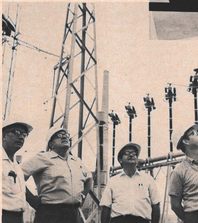
Progress on the 765KV switchyard occupies R. W. Palmer, W. C. Safford, Gilles Beaudoin and J. M. Kauffman, Jr., all members of the electrical section.
