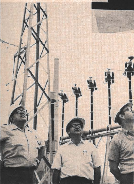
the 765KV switchyard occupies R. W. Palmer, W. C. Beaudoin and J. M. Kauffman, Jr., all members of the electrical section.
