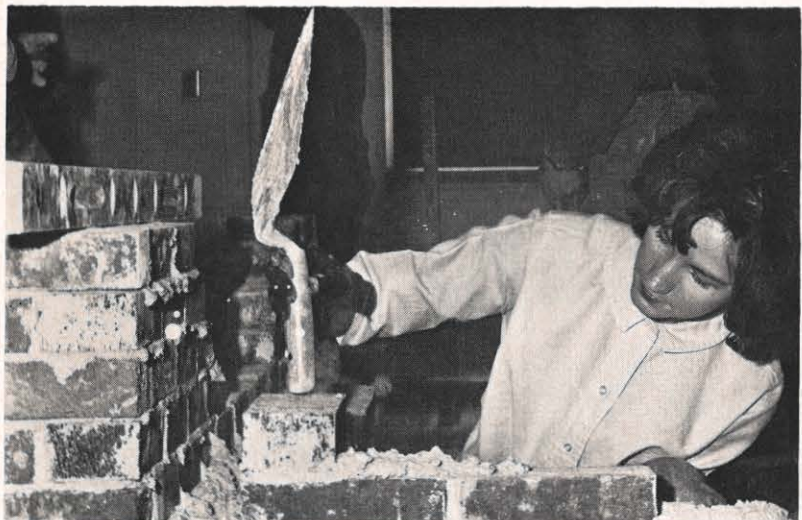
Brenda Aust taps a brick into place.
