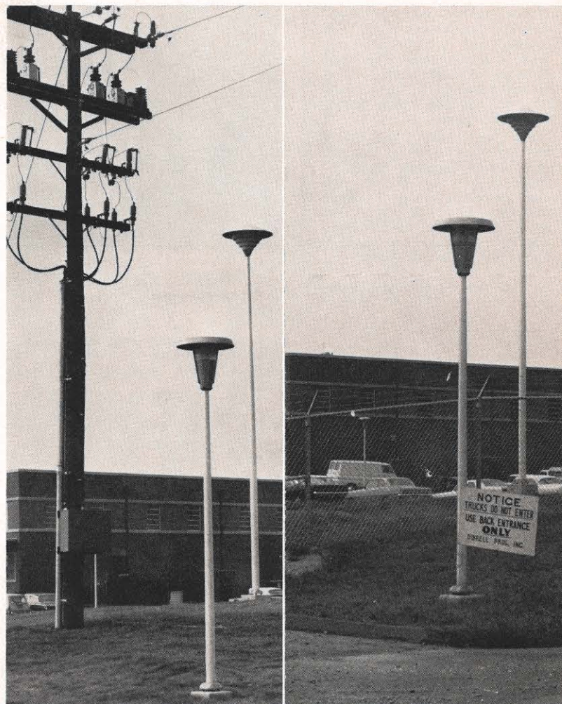
The before and after pictures here show how attention to aesthetics and reliable service can come together for everyone's good. The plant is Dibrell Brothers in the Danville Industrial Park. When Appalachian installed service, the primary arrangement at left was put in place. Adequate size metering equipment was not available to the plant at that time. Recently the company was in the area doing some work and was able to create an entirely new appearance for the entrance of the plant. A more efficient system for serving the plant was installed. The service went underground, the pole came down, and a clean, uncluttered view was created.
