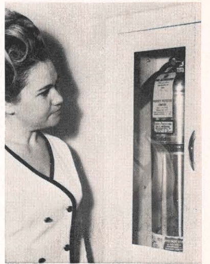
Knowing where fire extinguishers are and how to operate them is every employee's responsibility, as Patricia D. Cummings, personnel clerk sr., is doing here.
