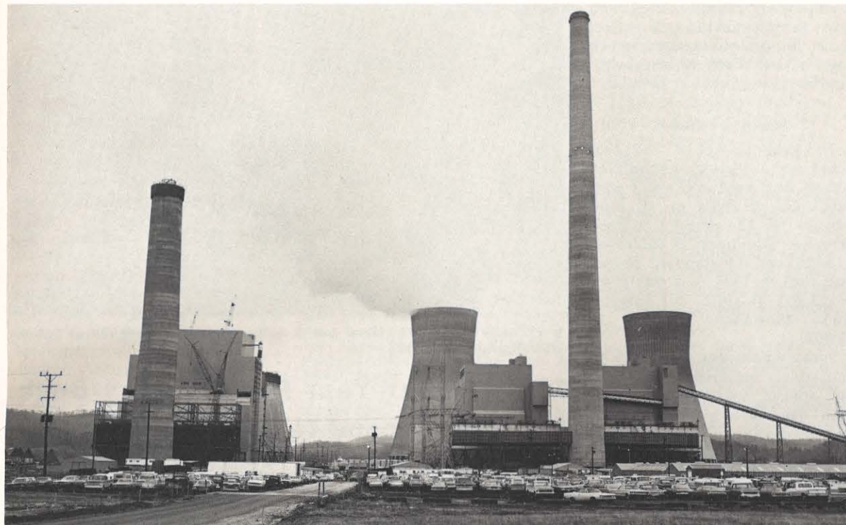
Higher and higher goes the Unit 3 stack (left) at John E. Amos Plant. The stack, a twin to the one for Units 1 and 2, will eventually reach 900 feet. Directly behind the Unit 3 building is the partially completed cooling tower.
