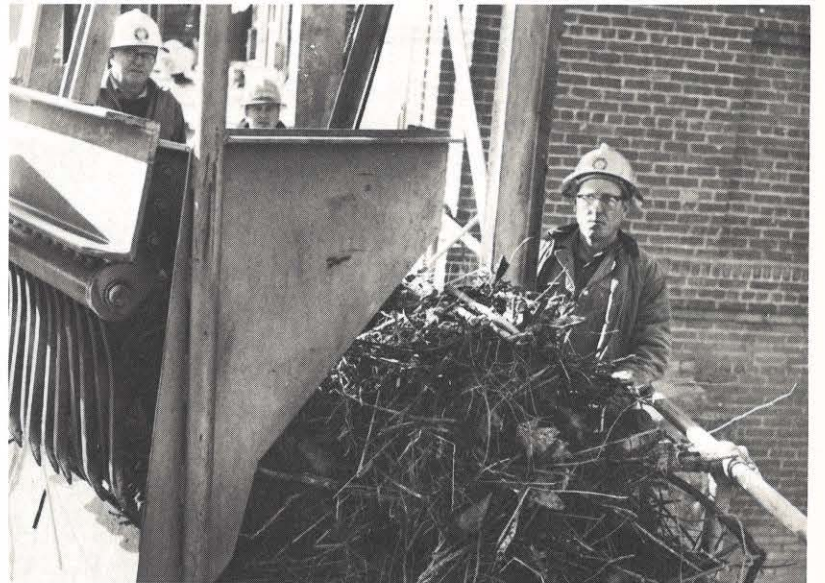
B. Q. Sharp (left), B. C. Litteral and D. E. Spraker unload trash cart at Byllesby after cleaning intake rakes.
