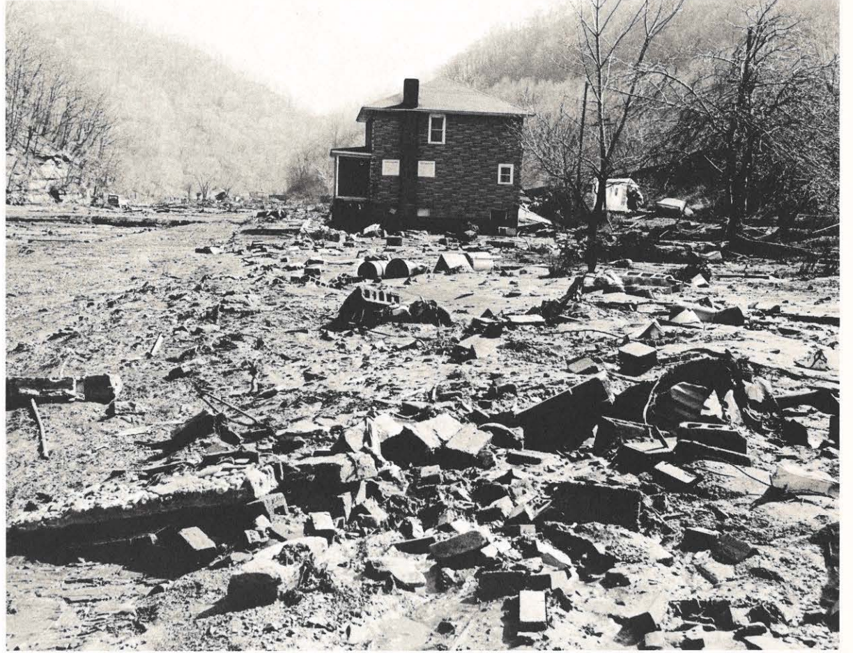
The Community of Lundale was one of the hardest hit. It is estimated that at least 100 homes were washed into and broken up by a bridge in the area. A smaller house (not visible in photo) washed into the back side of this one remaining home, inflicting severe damage. Part of a mobile home is visible at right. Photo courtesy Huntington Publishing Company.
