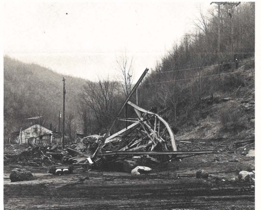
The onslaught of flood waters left Appalachian's Pardee switching station in shambles. The house in background was saved by being at the mouth of a side creek.
