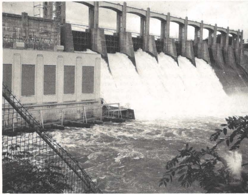
Water from the swollen New River rushes through the gates of Claytor Hydro.
