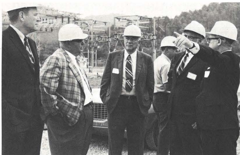
President Cook points out a feature in the 765-kv yard at Amos Plant. (L. to r.) Richard M. Dicke, AEP board member; Ray DeLancey, Amos Plant Construction; Richard G. Folsom and Walter O. Menge, AEP board members.
