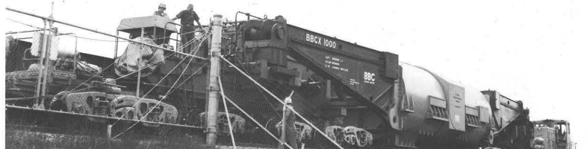
FROM ALPS TO AMOS — An intermediate pressure Brown-Boveri generator stator for Amos Unit 3 was lifted in place during November, ending a two month journey from Europe. One of two identical stators earmarked for Unit 3, this RH stator left Brown-Boveri Birrfield factory in Switzerland on September 9 by rail, routed to Hamburg, West Germany. From there it was sent to New Orleans by ship and was transported from New Orleans to Amos by a special schnabel car, designed in Europe especially for this purpose. This schnabel car is a 20-axle car, weighing approximately 418,000 pounds. The generator was bolted to the transporting apparatus, which measured 155 feet from end to end. Because of the weight and length of this shipment, engineers from Brown-Boveri accompanied the car to its destination. On long curves the shipment would normally be moving inside. In these instances, the engineers used special mechanical devices to shift the unit and move the center of gravity to prevent it from turning over on the inside curves. The stator is approximately 12.5 feet in diameter and 41 feet long, including end bells.
