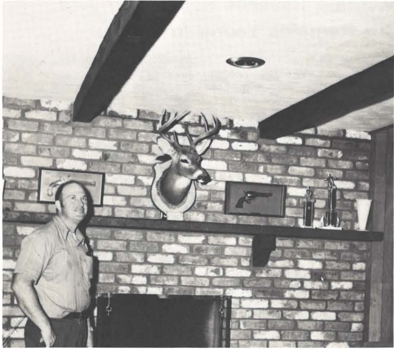
Tom Young hewed the beams in this recreation room from discarded utility poles.
