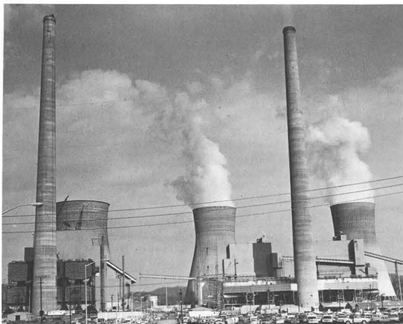
Unit 3 (left) at John E. Amos Plant is nearing completion.
