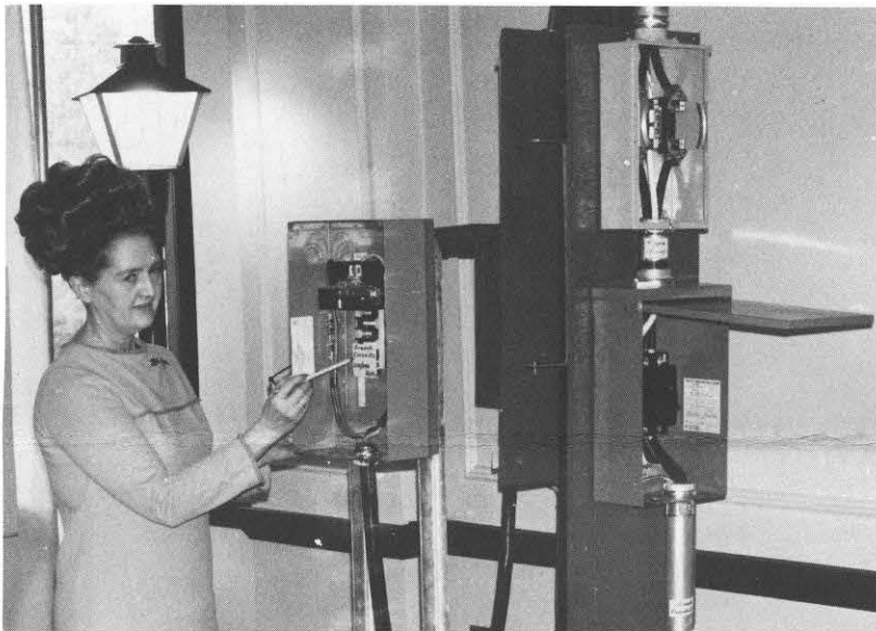
In an effort to speed service installations to mobile home customers, the Logan-Williamson Division T&D Department designed and built several mock installations which are located at various points throughout the division for customer inspection. These mock-ups, subject of an operations improvement proposal, were the idea of Fred E. Varney, Williamson line and station supervisor. The mock-ups cover any particular situation which might apply
