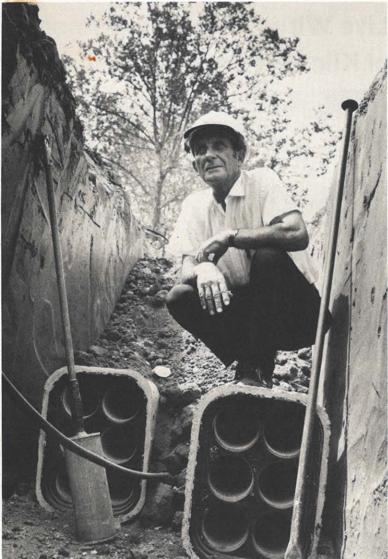
A proposal describing the use of precast conduit and manholes submitted by Huntington Electrical Engineer Joe Kovich was judged best in the division category.
