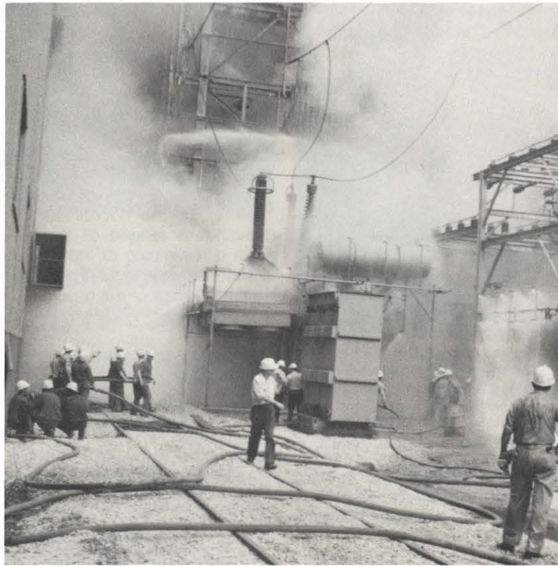
The fire brigade at Amos Plant rolls into action following an explosion in the ASEA main transformer bank on Unit 2.
