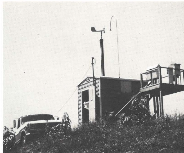
AEP System air monitoring station near John E. Amos Plant.
