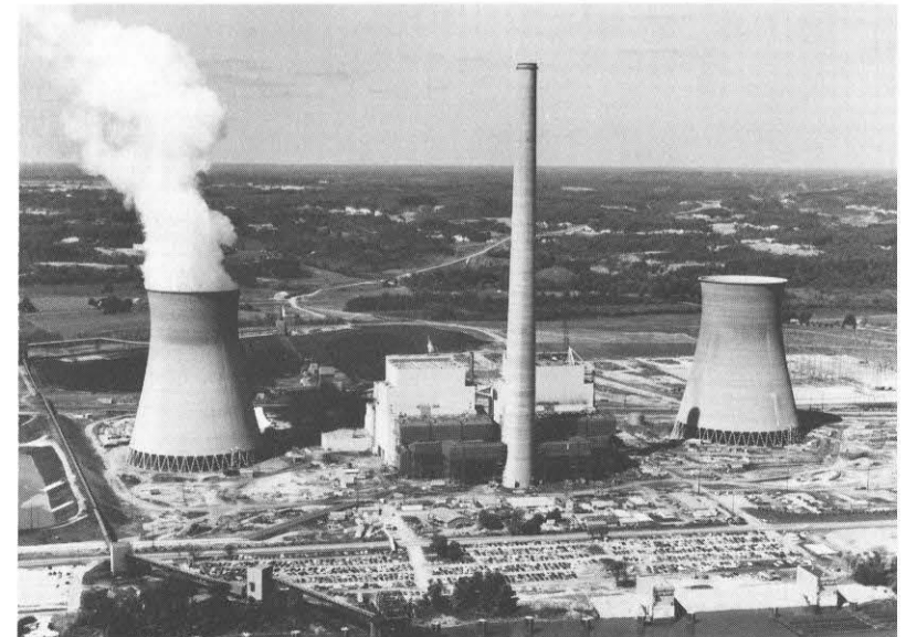
Environmental control equipment is much in evidence at the General James M. Gavin generating station. At left and right are 492-foot cooling towers. Steam rises from the tower for Unit 1 which is now in commercial operation. The 1,103-foot stack disperses into the upper atmosphere any gases emitted from the plant. At the base of the stack are electrostatic precipitators designed to remove 99.7 per cent of the ash particles resulting from the burning of coal. These facilities represent about $64-million of the plant's total estimated cost of approximately $585-million.
