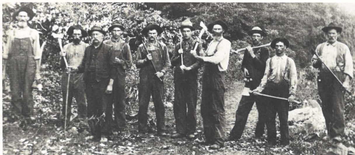
Members of the original crew who cut brush and timber for the construction of Byllesby dam were (from left) Bud Harmon, Cage Porter, Buck Shelton, E. C. Bryant, Joe Bryant, Elmer Bryant, Meredith Burnett, Steve Landreth, John Henry Frazier and Floyd Robinson.
