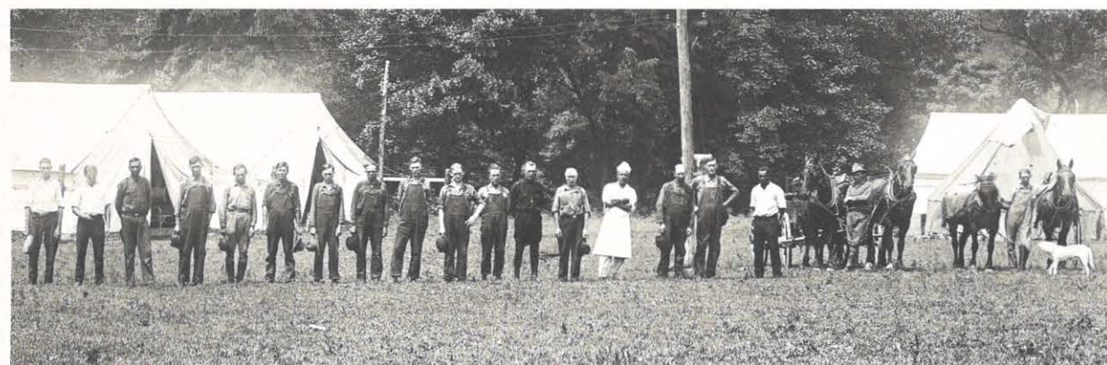
This is how Camp Tenderfoot at Nighbert, W. Va., looked in 1924. This was the construction camp of Kentucky and West Virginia Power Company for the building of a line from Dehue to Earling.
