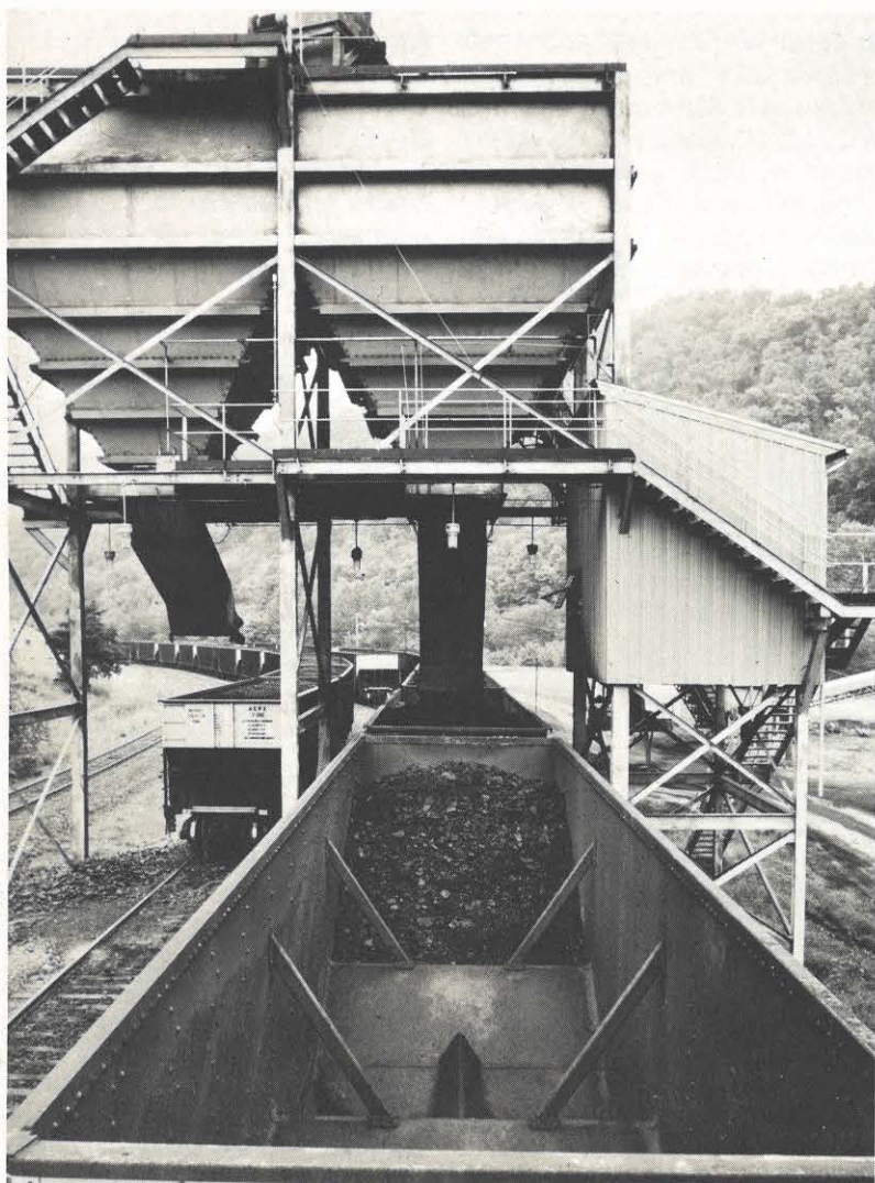
Julian Mine, Southern Appalachian Coal Company
