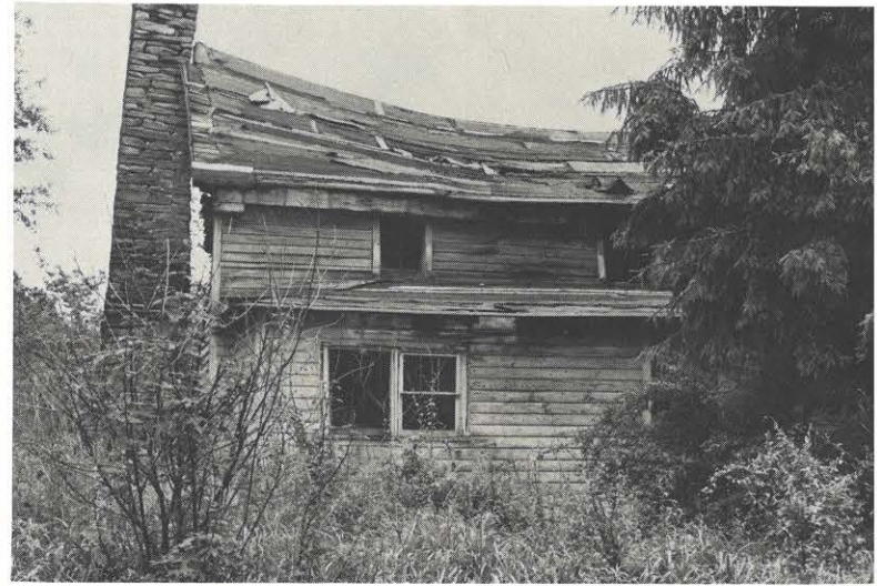
This house, which once belonged to Preacher Hatfield, stands on the election grounds where Ellison Hatfield was stabbed.
