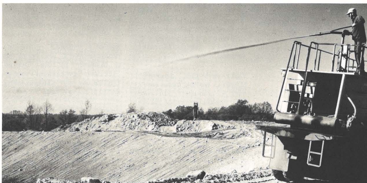
Reclamation of surface-mined land, Cedar Coal Company
