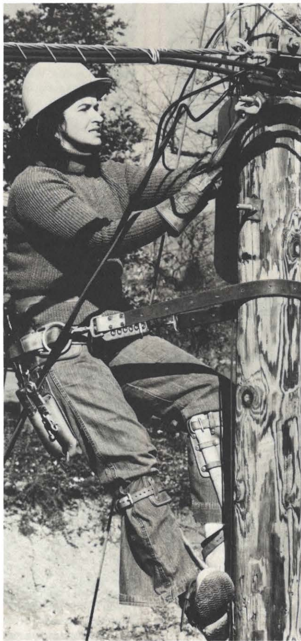
Mary Slocum, lineman, Roanoke
