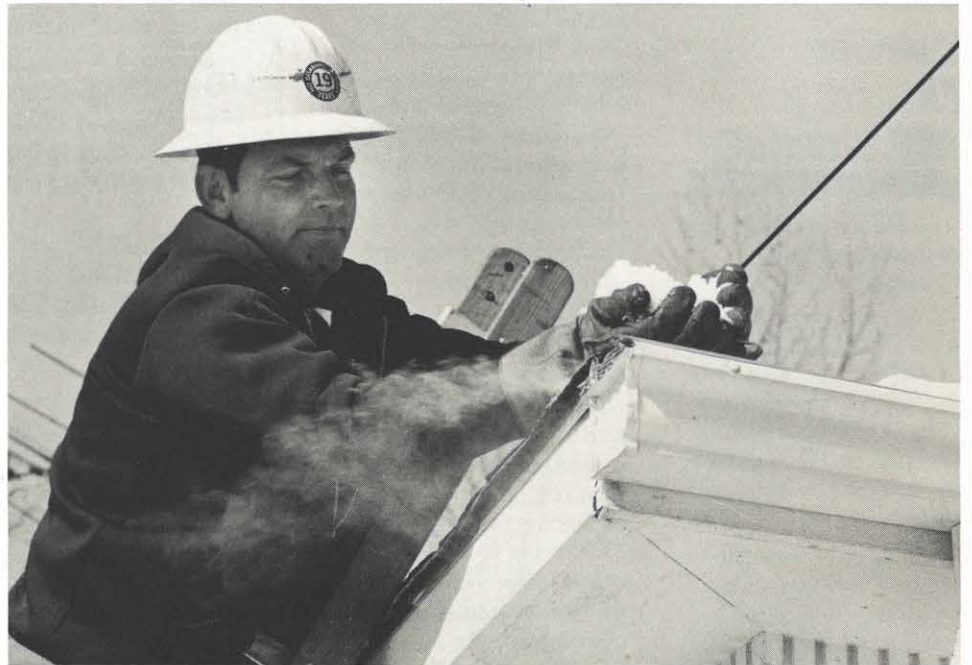
Glen Hicks extinguishes the fire on the roof of a customer's house with snow.
