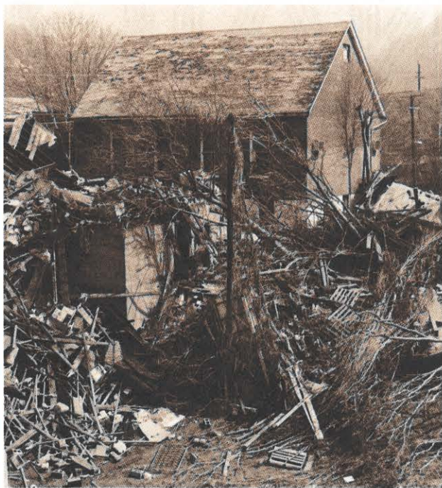
Typical of the devastation throughout flooded area.
