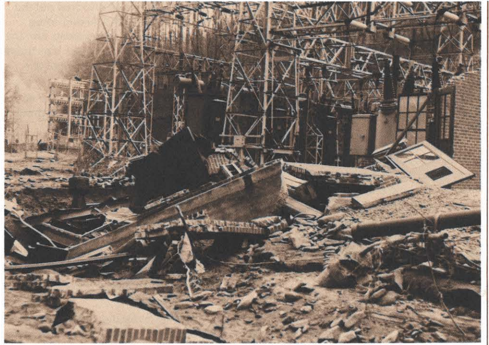
All that remains of the control building at the Grundy Substation.
