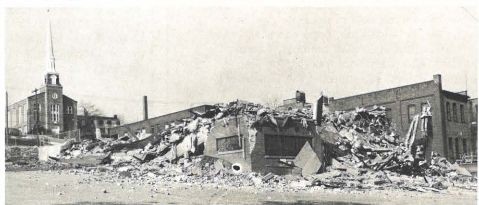
Ready for the bulldozers
