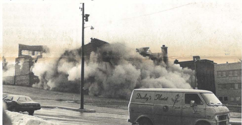
Building sags as supports are blasted apart
